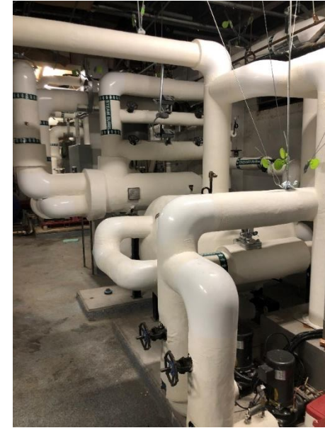
Dennis Building (after)
